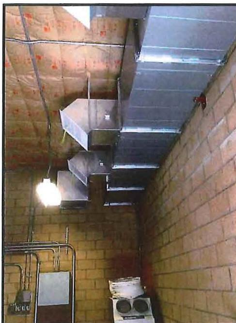
Installed ceiling insulation and AC air ducting
